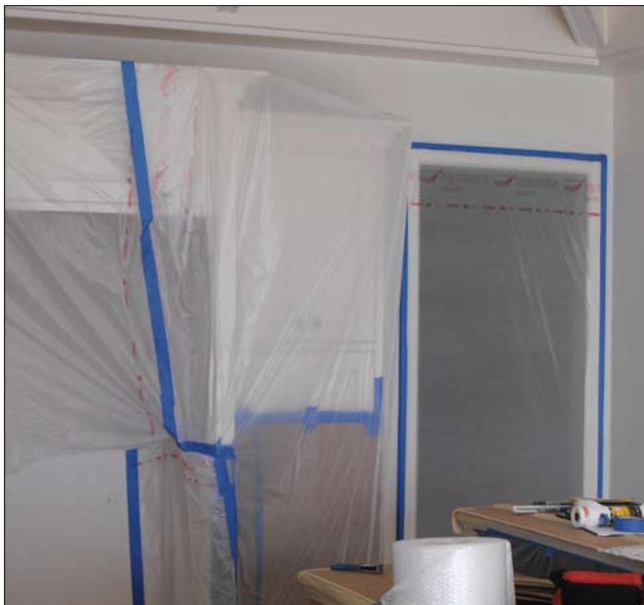
**Cabinet Protection - The cabinets in this home were covered and sealed to protect them from dust, debris and the elements during renovation of that portion of the home.**
